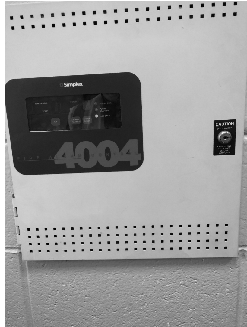
EXISTING CORROSION CONTROL FACILITY FIRE ALARM PANEL
